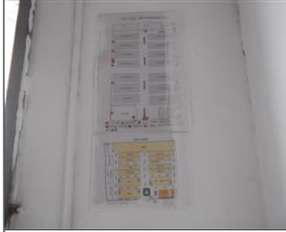
Photo of fire safety equipment Evacuation map.JPG
