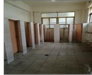
Photo of the sanitary facilities Toilet.jpg
